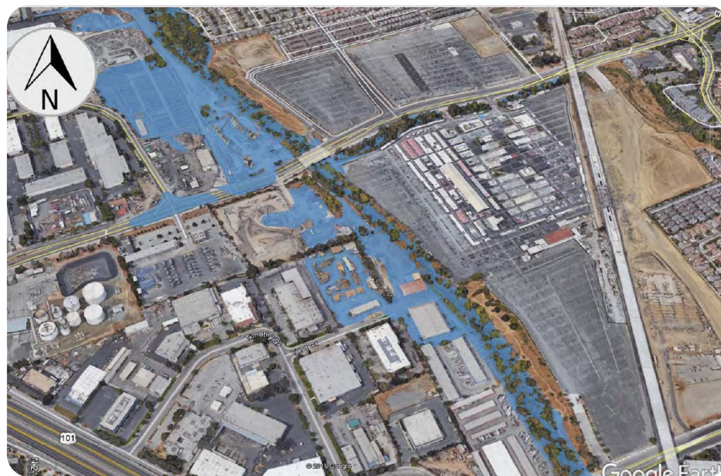
Figure 3. Coyote Creek flooding on February 2017 at Berryessa Rd. Source: SCVWD 2017 Flooding Report
