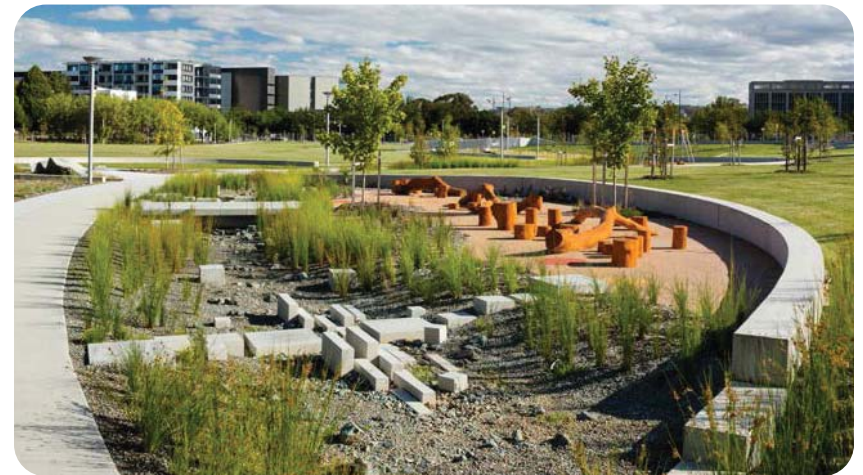
Figure 40. Integrated treatment and ponding area in Hassett Park in Campbell, Australia. Source: City of San José, GSI Plan
