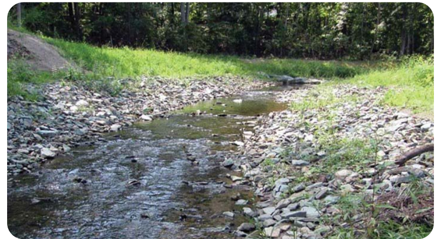
Figure 23. Meadow Creek Stream Restoration. The images shows the degraded creek and eroded bank before restoration (top); the bottom image shows the restored stream with wider and vegetated riparian. Source: www.landscapeperformance.org
