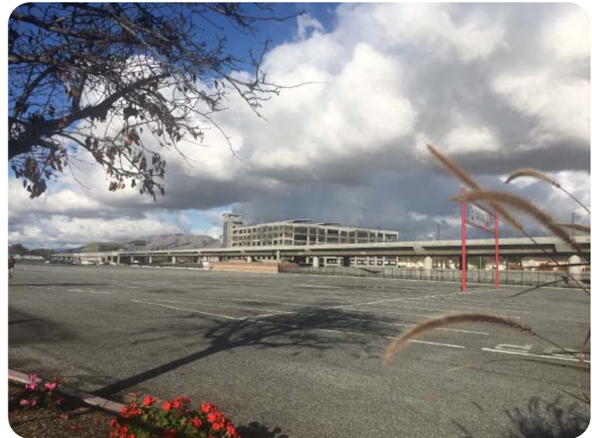
Figure 14. Existing Flea Market parking lot near Mabury Rd. Behind is the BART station and its parking garage. Photo by the author.
