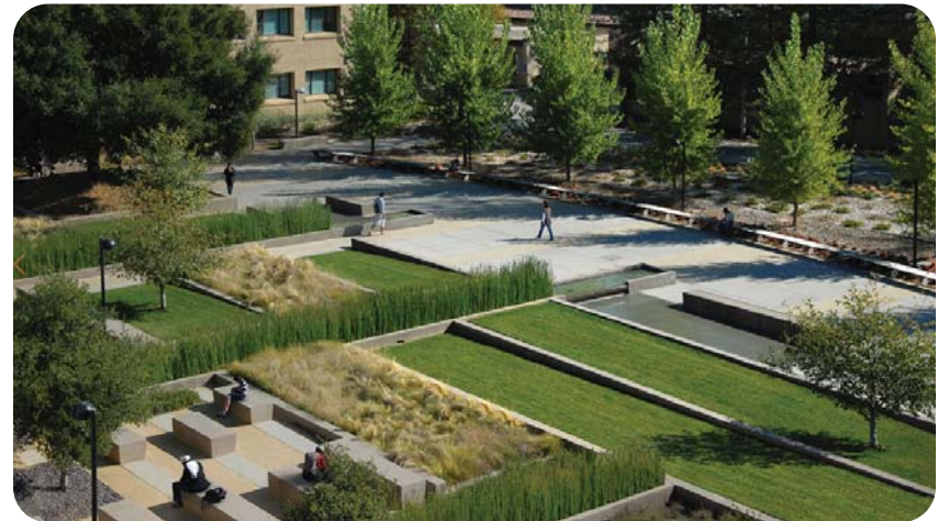
Figure 42. De Anza College - Media and Learning Center, Cupertino, CA. Native vegetation and the bio-filtration system treats and stores stormwater runoff. Source: Office of Cheryl Barton (O|CB)
