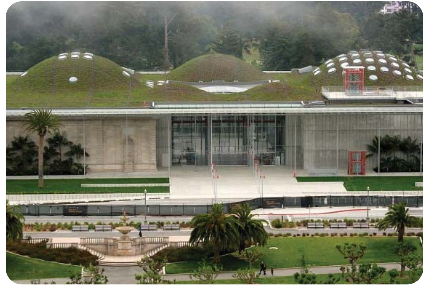
Figure 41. Green roof in the Academy of Science in San Francisco, CA. Source: www.ecourbanhub.com
