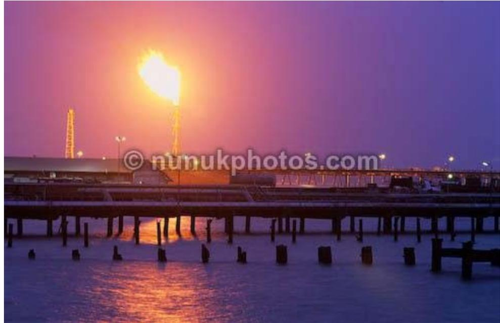
*Refineries and chemical plants are equipped with these to burn off waste, especially during accidents. In this case, the accidental release gasses are routed to flare to be burned off.*
