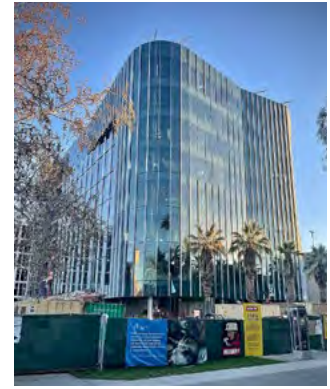
Interdisciplinary Sciences Building - under construction and part of the goal to Rebuild and Renew
